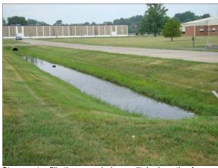
Storm water fills the open drainage ditch along the Armory Road right-of-way, evidence of inadequate drainage facilities.
